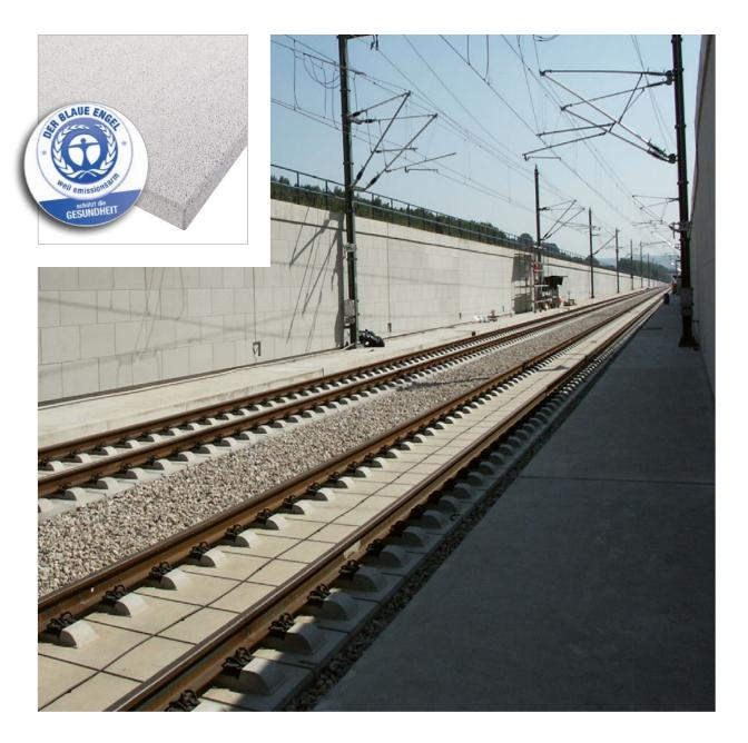
pinta phonestop V sets new design trends: inside or out. The basic material used for this acoustically highly effective, and purely mineral absorber is expanded glass granulate.
